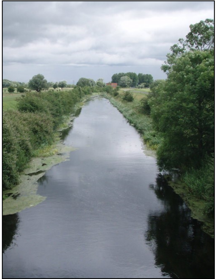
A view of the Maxey Cut, which runs between Peterborough and Market Deeping. The cut was originally created as a flood relief channel for the River Welland.
