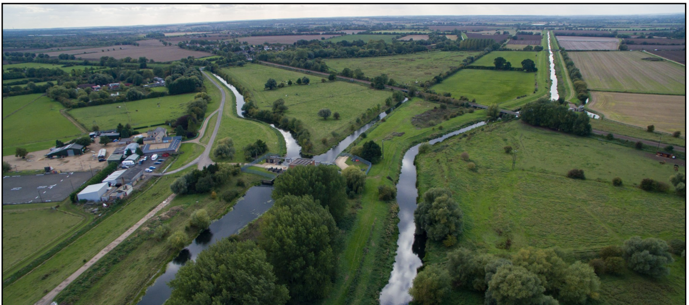
This photo by Nicholas Jackson shows the confluence between the River Welland, Maxey Cut, Folly River and South Drain just outside Peakirk, clearly demonstrating why control of the water levels is so important when considering new development. It also shows the recently upgraded Spalding-to-Peterborough railway, cutting across the picture.
