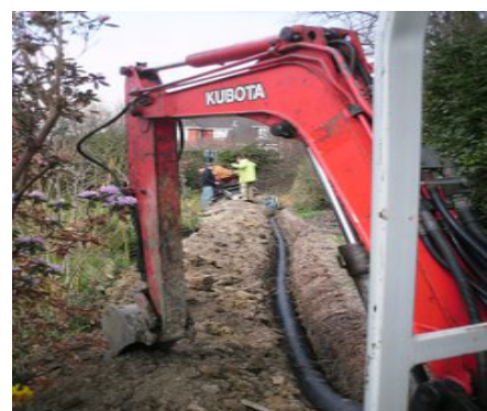
Laying a district heating pipe, Hoathly Hill, High Weald
